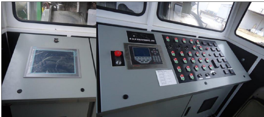
Figure 4: The control panel for the semi-automatic operation of the RAR production plant
