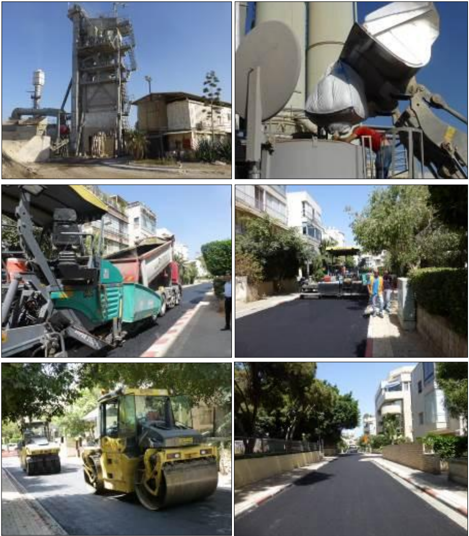
Figure 10: Photographs describing the production batch mixing plant, filling the SMA fibres bin with RAR, laying, and compaction with steel and pneumatic rollers. A day work on September 17, 2014 (an ability-proof road test)
