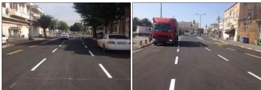
Figure 13: Photographs showing the surface condition of sub-section A in Salame Street on the day following construction (November 12, 2014)
