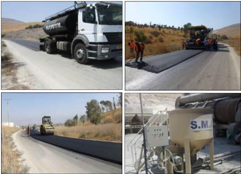
Figure 5: Photographs describing the application of Tack-coat, laying and compaction, and RAR feeder during the October 12 th 2012 road test
