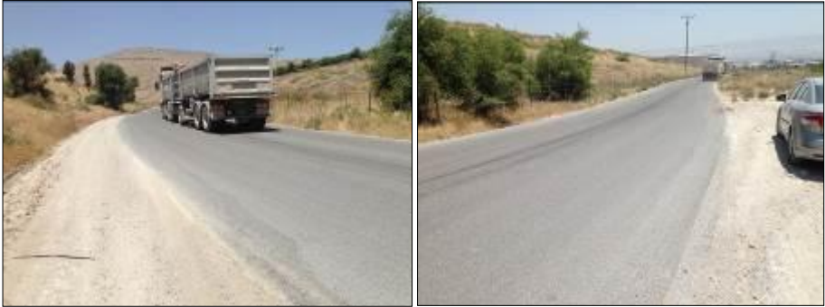
Figure 9. Pavement and top RAR Asphalt Rubber layer after two years from construction date
