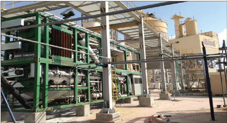
Figure 3: RAR production plant installed and operated in the Dimona Isreal
