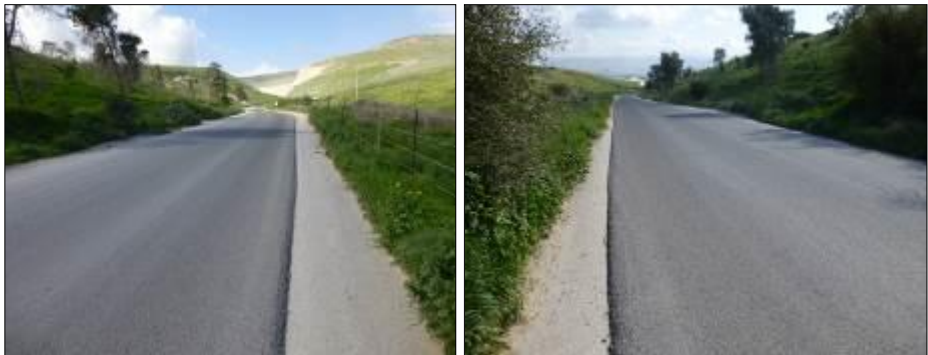
Figure 8. Pavement and top RAR Asphalt Rubber layer after four months from construction date
