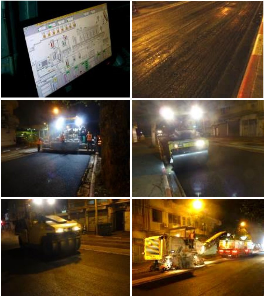
Figure 12: Photographs describing the mixing plant control panel, tack coated surface after milling, laying, compaction with steel and pneumatic rollers, and milling the opposite direction lanes while loading an empty asphalt mix truck. A night work on sub-section A in Salame Street, November 10/11, 2014
